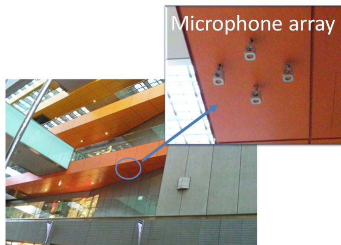
Fig. 1 Microphone array utilized to collect environmental sounds at a Galleria.
